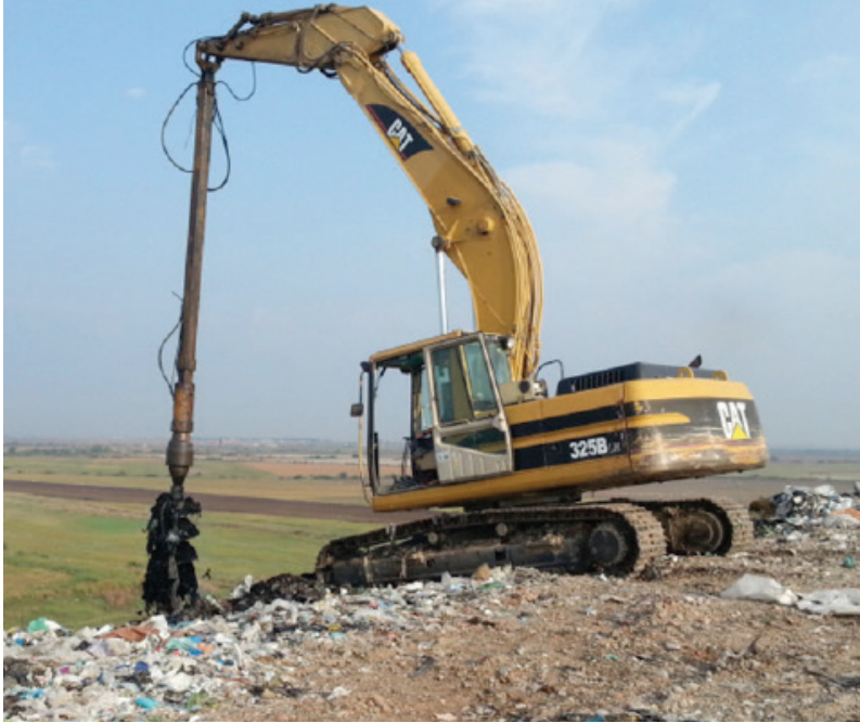
Drilling of degas wells, Arad, 2014.
